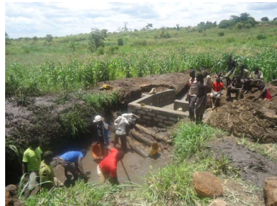
Spring well under construction
